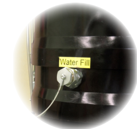
Water fill connection backflushes dispersion screen
